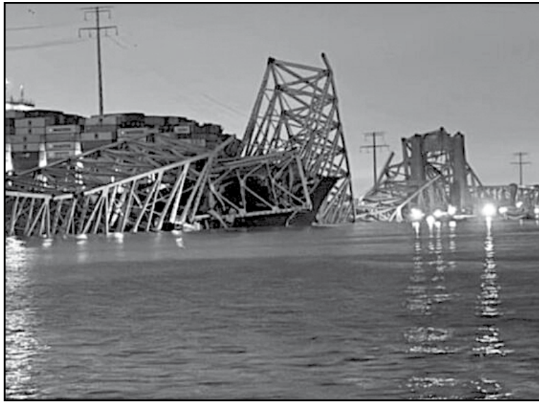
Francis Scott Key Bridge in Baltimore, Maryland.
